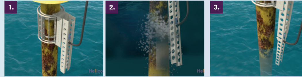
1. Installation of the Helicoid Surface Preparation System
