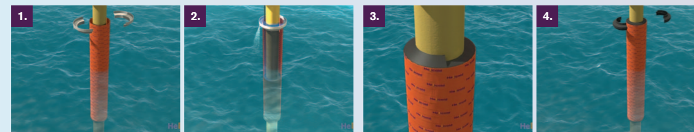
1. "Grout collector" is placed to prevent spillage
